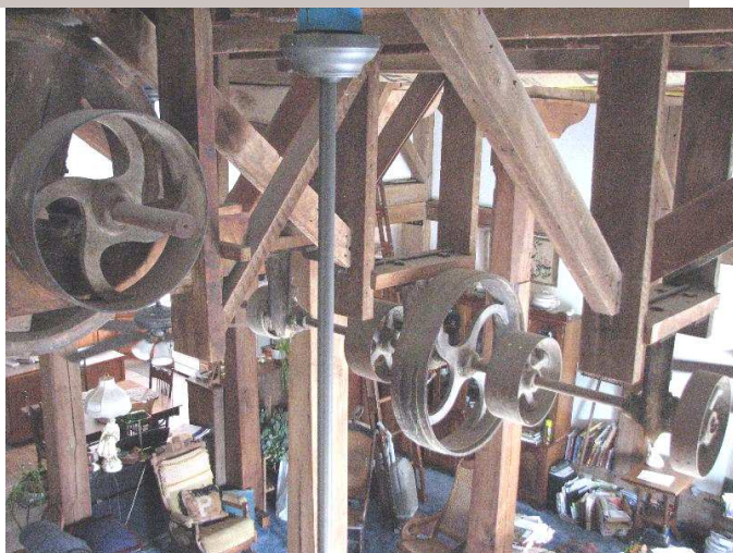
The Shell Rock mill equipment remains at ceiling level with the living room/kitchen at floor level.
