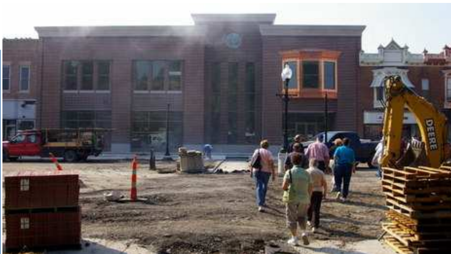
Heading to the "under-construction" Public Library in Washington, IA.
